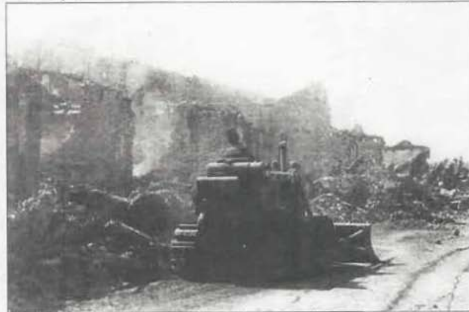
EOH3 Antonio of Seabee Team 1011 clears away bomb damaged structures in Vinh Long, Vinh Long Province; the aftermath of TET '68
