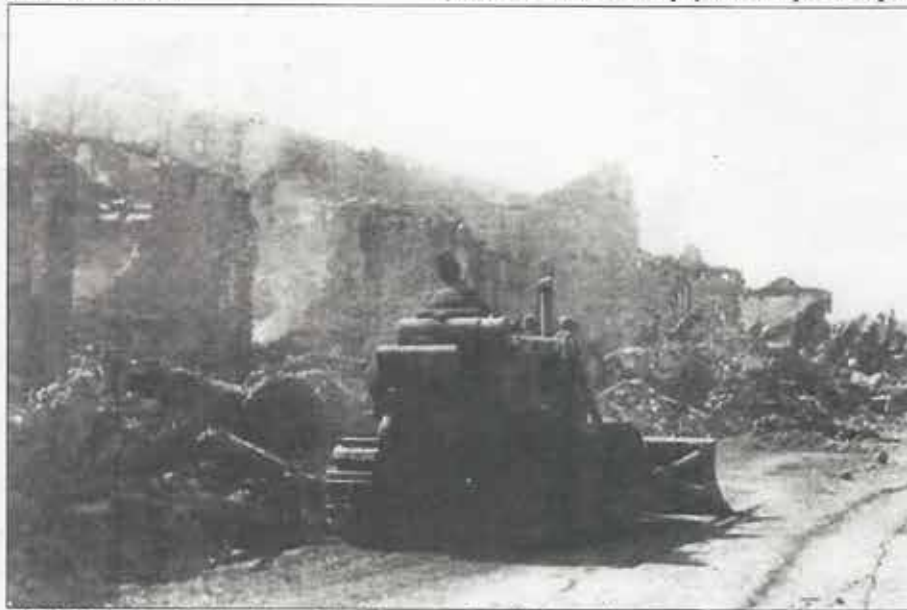
EOH3 Antonio of Seabee Team 1011 clears away bomb damaged structures in Vinh Long, Vinh Long Province; the aftermath of TET '68
